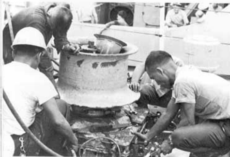
Port Anchor Windless. This was Excedrin headache number 39.
