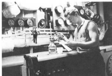
Ray Erskins takes water samples in the Boiler Room.
